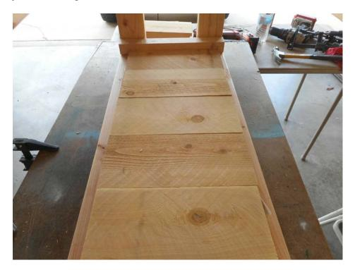
Please notice there is only one nail top and bottom. this is to allow the cedar to expand and contract depending on moisture content, and als very important. you need to center them top to bottom. There should be gaps to allow for drainage.
